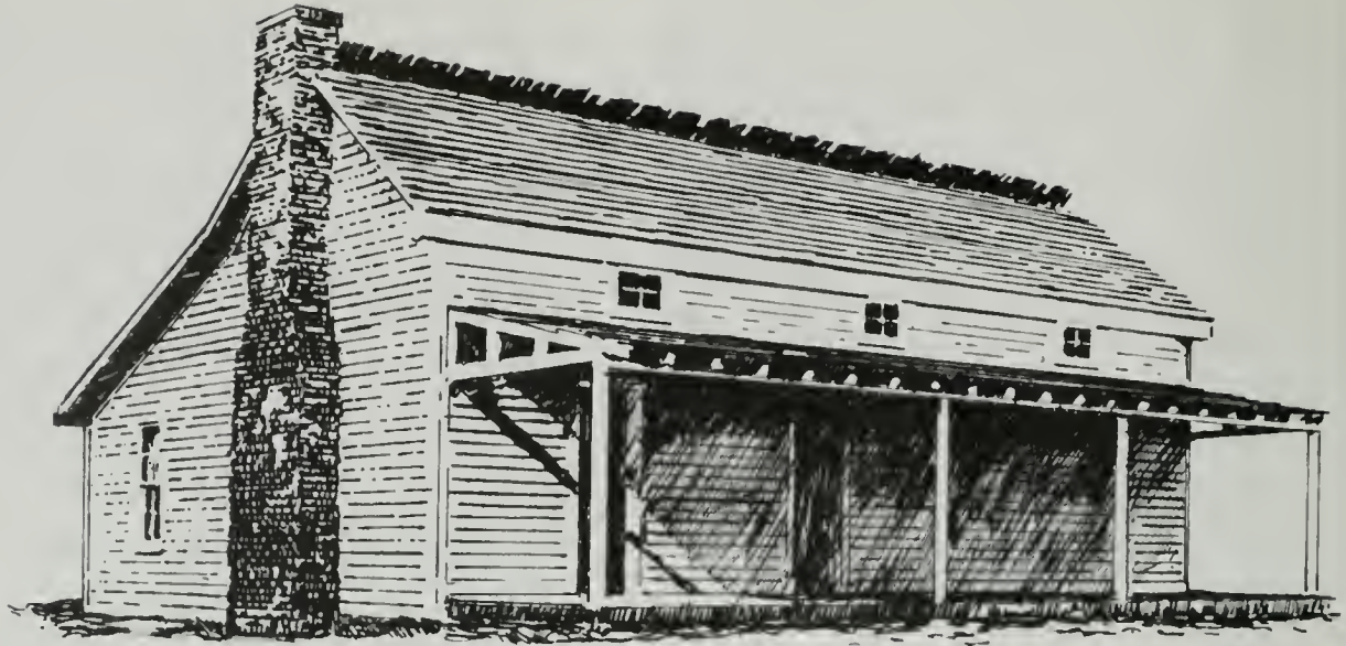
LOG HOUSE WITH CLAPBOARD SIDING
